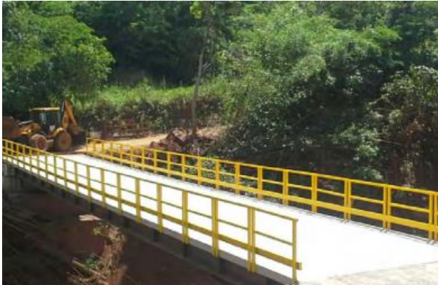
Infrastructure reconstruction, Mariana
